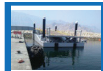
25m RoRo Link Span
